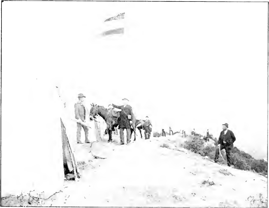
Breaking Ground for the Cable Road Division on the Site of the Mountain House
